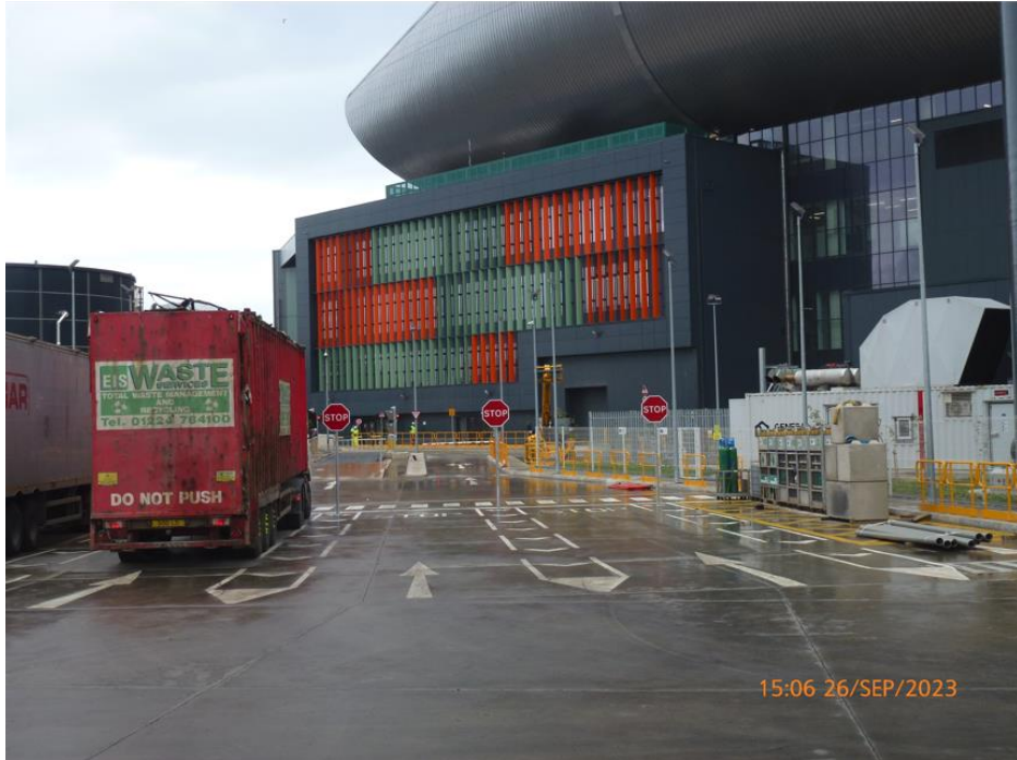
Staff parking area looking towards office block
